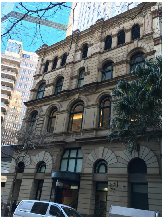
Figure 3.4 View of the former Coal Exchange Chamber facade. (Source: GML Heritage, August 2019)
